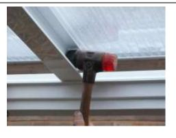
Do not secure the main glazing bars or last edge glazing bar at this stage.
