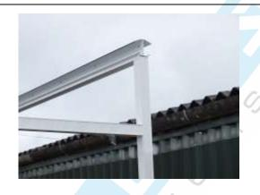
Glazing Bar assemblies (Edge and Main Glazing Bars with Main Glazing Bar End caps fitted). Fit the Edge Glazing bar and secure in position. Working from one end of the canopy fit one roof panel followed by one Main Glazing Bar assembly alternatively until the last edge glazing bar has been installed in position.
