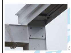
Secure the Eaves/Gutter to the Supporting Posts via the the Supporting Post brackets.
