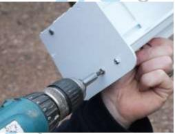
The (4) holes in the Eaves/Gutter End Plate align with the (4) screw ports in the Eaves/Gutter.
