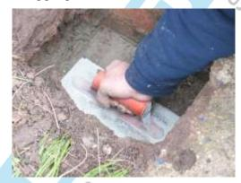
It is highly recommended that the concrete pads are made to be level with each other. This will save a huge amount of time later when levelling the canopy frame components. Therefore. It is worth getting this right.
