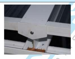
11 Secure the Main Glazing Bars in position at the Wall-Plate and the Eaves/Gutter.
