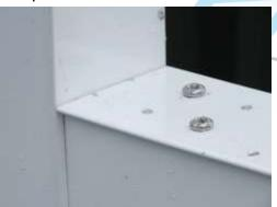
Fix the Tie-Bar to the Supporting Post/Tie-Bar Bracket Assemblies by driving the No.12 x 13 Self-Tapping screws through the Tie-Bar into the Tie-Bar bracket using the Drill Driver and PH3 Driver Bit.
