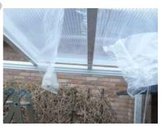
This Main Glazing Bar must be positioned before securing with the Self-Tapping Screws.
