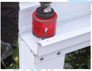
Please note that in this picture the Eaves/Gutter end-Plate has been removed to show the HoleSaw position.
