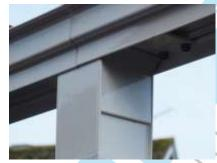
Apply Flashband to internal join of the (2) Eaves/Gutters. This is to seal the join in the gutter.
