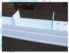
In order that (1) Bracket for each Supporting Post is secured in position you will need to measure where the Posts will be located along the Eaves/Gutter and mark these positions before securing these single Brackets in position on the Eaves/Gutter.
