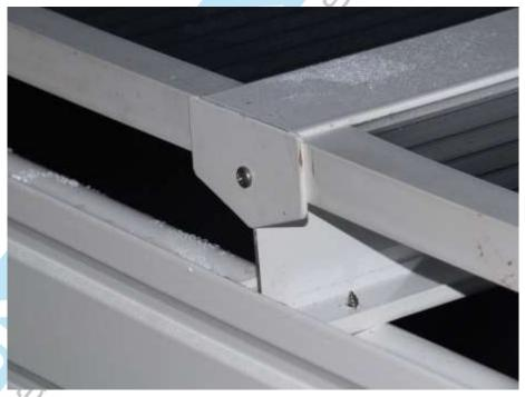
Slide the Sheet Closure onto the end of the Roof Panel.
