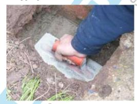
It is highly recommended that the concrete pads are made to be level with each other. This will save a huge amount of time later when levelling the canopy frame components. Therefore. It is worth getting this right.
