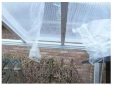
This Main Glazing Bar must be positioned before securing with the Self-Tapping Screws.
